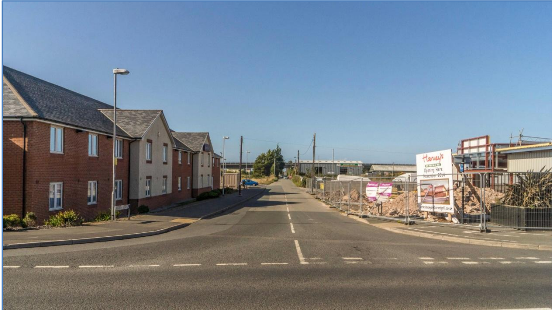
7.3 Photo 7 View along Marsh Road from T-junction with Station Road (September 2014)
